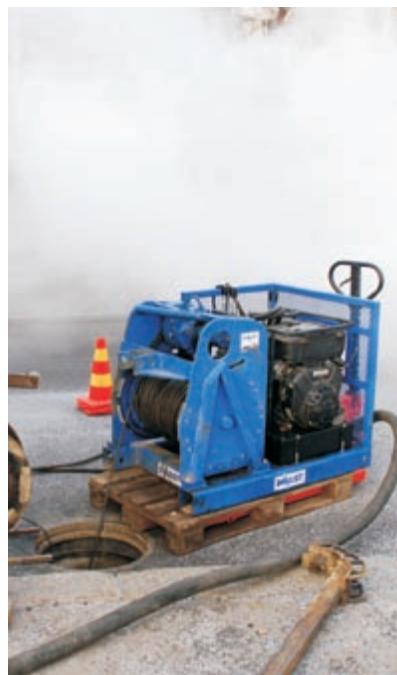
A 10 ton HVY doing pipe lining at a pipeline renovating site. Pulling the tube from one manhole to another takes a few minutes.
